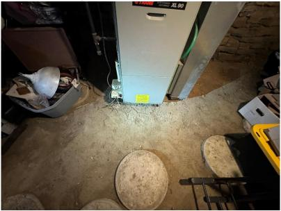
5) Foundation walls (in areas that have foundation) are stone, permitting water intrusion. French drain system is required to be installed and tied into city storm water system.
