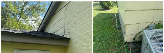
7) The paint on the brick is failing and chipping. Additionally, the brick shows signs of efflorescence and mortar failure. The paint needs to be stripped, the brick acidwashed and the areas of failing mortar tuck-pointed.
