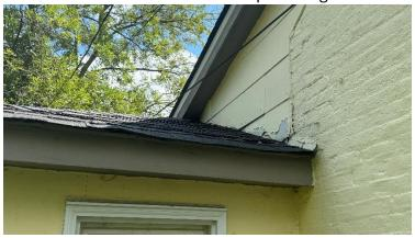
5) The soffits, rake boards and gutter boards are all failing and require replacement.
